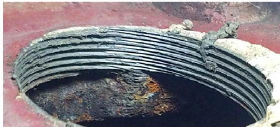
16) **Dry Pipe Seal Welded To Front Tubesheet**
