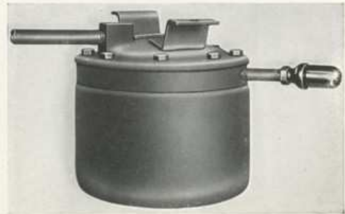
Fig. 3. Photographic View of the Type "C" Signal Valve and the Signal Whistle
